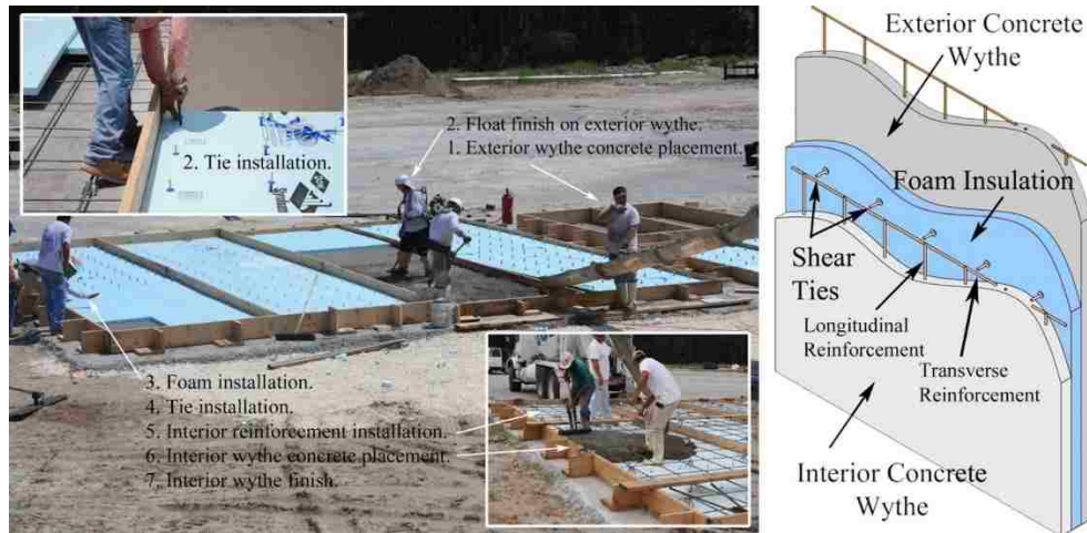
Figure 1: Insulated wall panel construction and configuration
